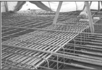
Figura 7. Barre e staffe in GFRP
